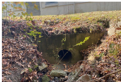
Figure 4-5. An outfall during a dry weather screening assessment
